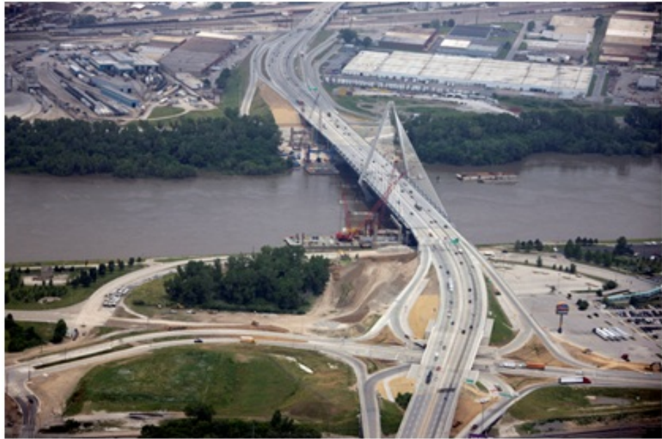
Latest aerial view of the project taken this month.
