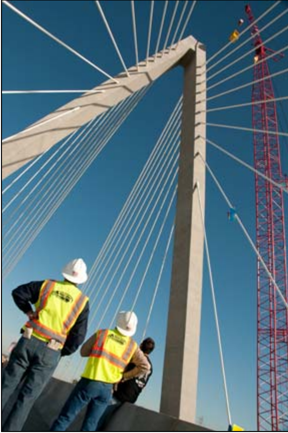
Onward and upward: cables radiate from the center pylon of the new, Christopher S. Bond Bridge.
